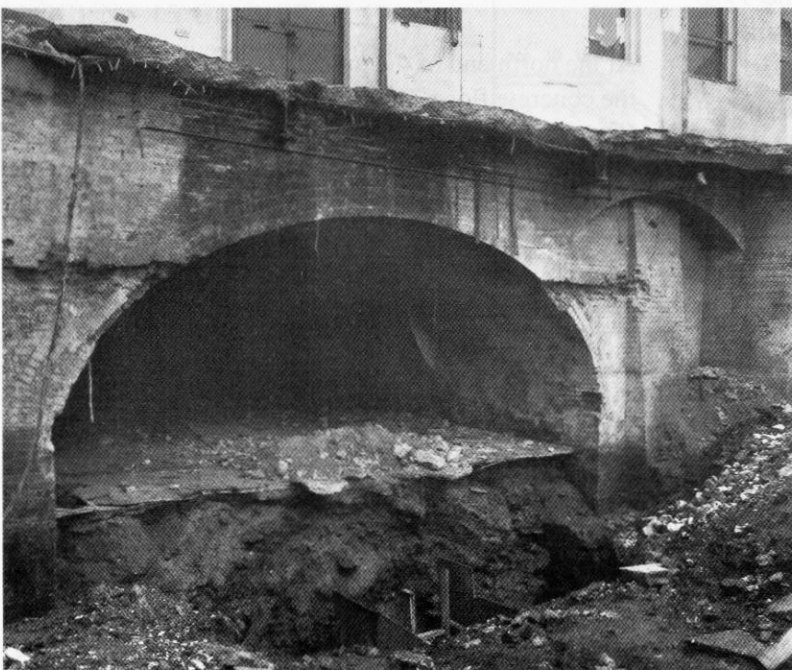
The Southern Portal excavated during the construction of Robinscroft Mews in 1987. Photo by Nick Catford
